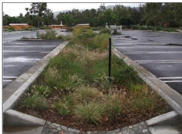
Example of bioswale within a parking lot.
