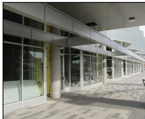
Example of anti-reflective glass storefront.
