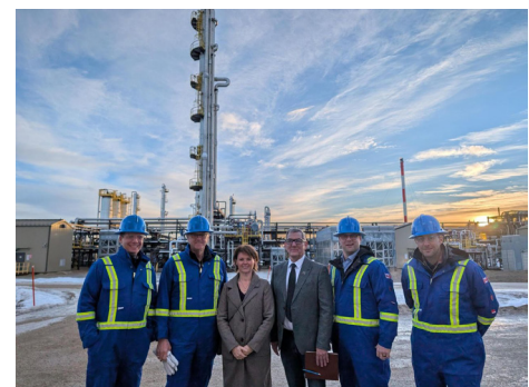
AltaGas Pipestone II facility began operations December 7, 2025
