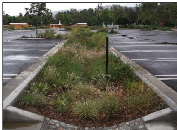
Example of bioswale within a parking lot.
