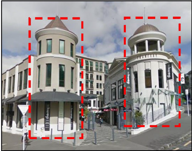
Example of enhanced architectural elements at entrance.
