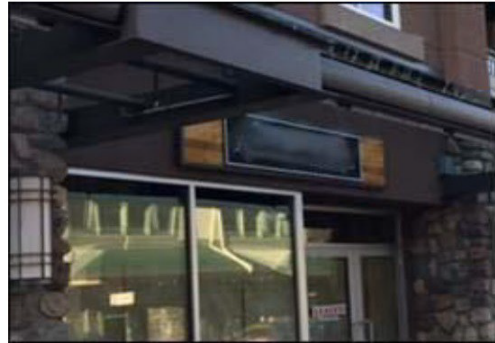
Example of fascia sign.
